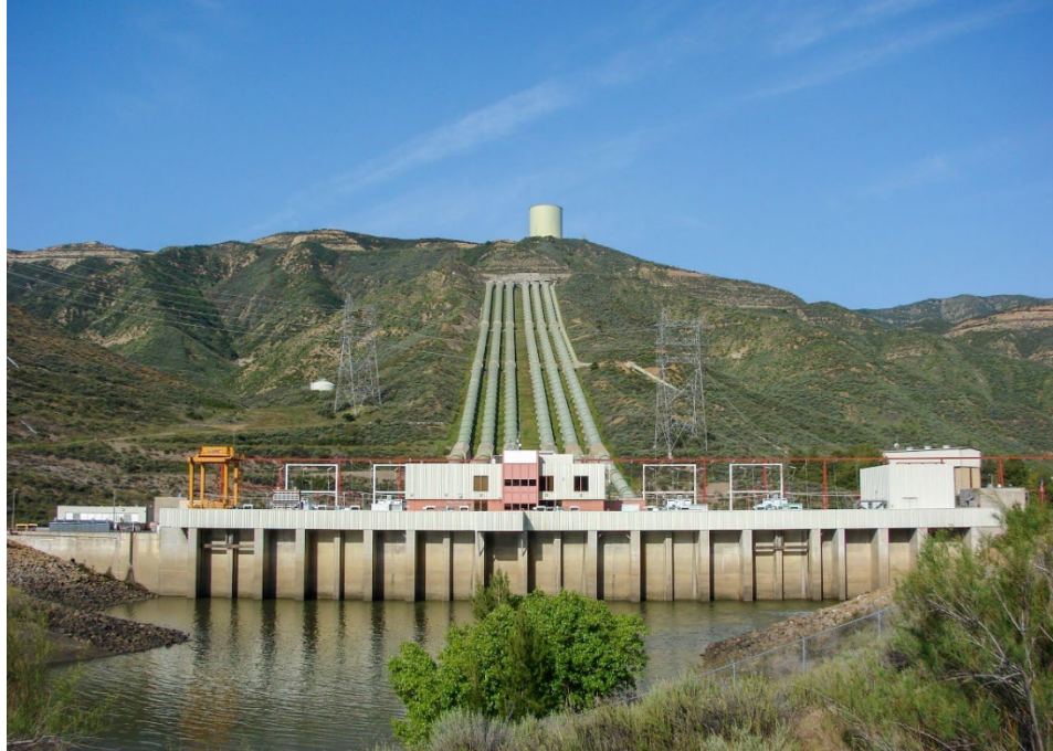
Picture of the Castaic Power Plant taken by a power plant worker facing east from the Elderberry Forebay. By Sirbatch at English Wikipedia, CC BY-SA 3.0, https://commons.wikimedia.org/w/index.php?curid=86486796
